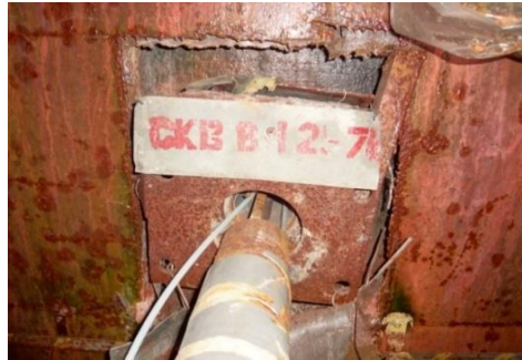
Sampling in borehole
