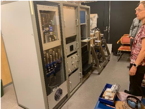
Installation in Stockholm
