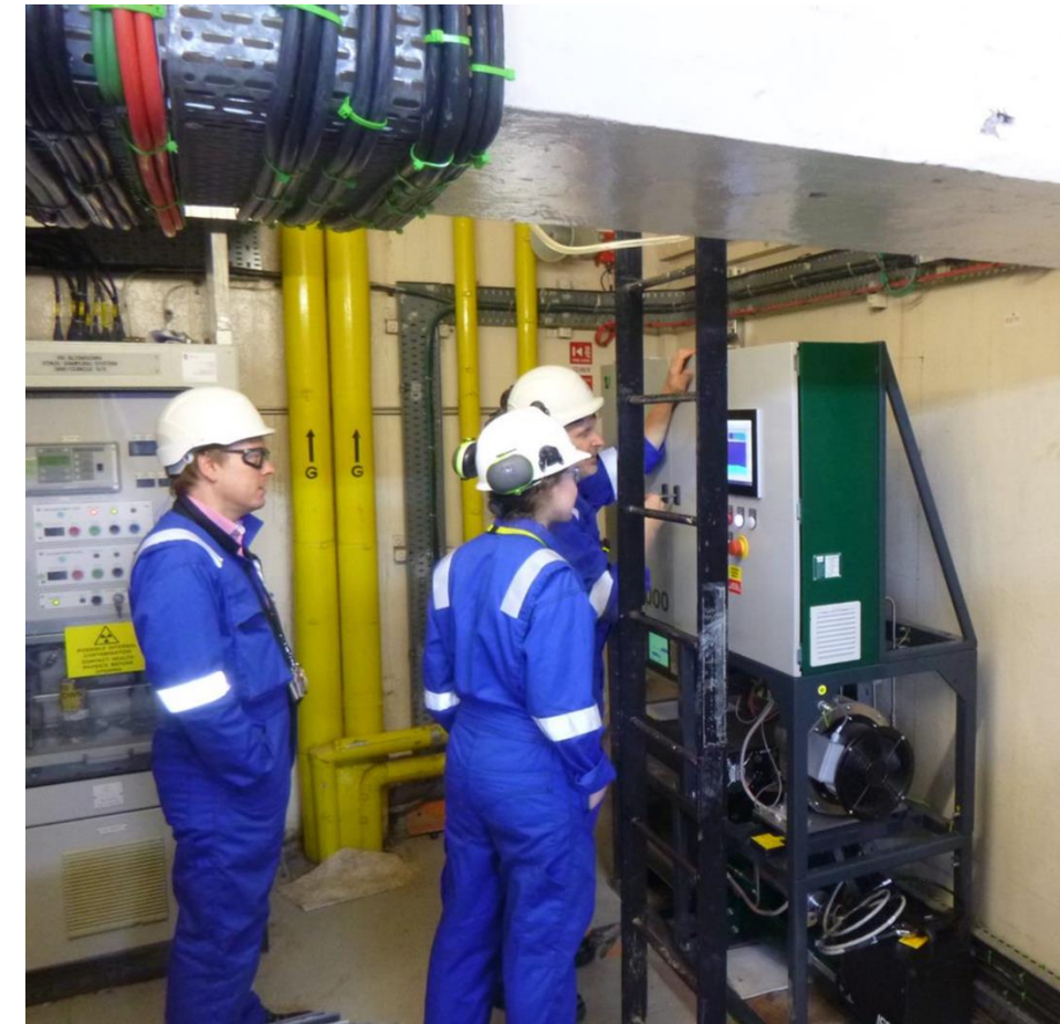
VF Nuclear High-purity germanium (HPGe) detector installed at Hartlepool
